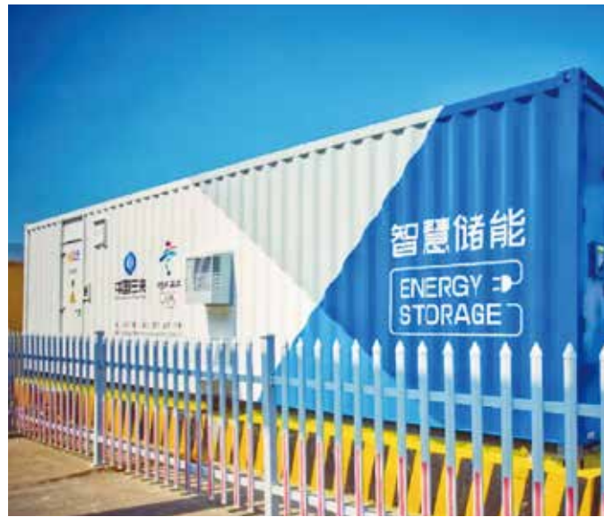
Siyang Wood Industry Park Photovoltaic Storage and Charging Project Project scale: 6MW photovoltaic + 2MW/8MWh Project location: Suqian, Jiangsu
